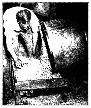
FIGURE 35 Multifacture of Globe Torpedoes Removing the moist spheres from the tumbling barrel. (Courtesy National Fireworks Company and the Boston Globe)
